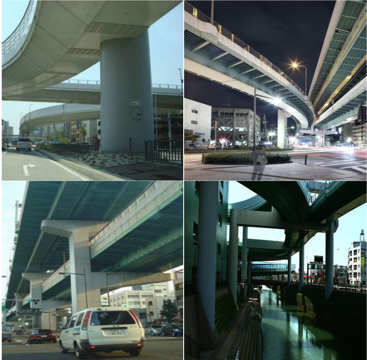
Fig. 1.1. In-service Steel Bridge Piers (Courtesy of Google).
